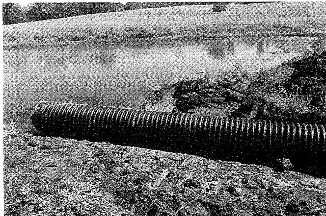
Figure 2: Installation of culvert on sedimentation pond North of Willow Creek.
